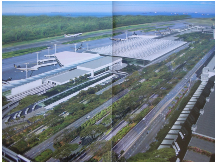
Overall view of the Terminal 3 after finished
