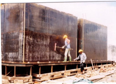
Precast segments at different stage of process
