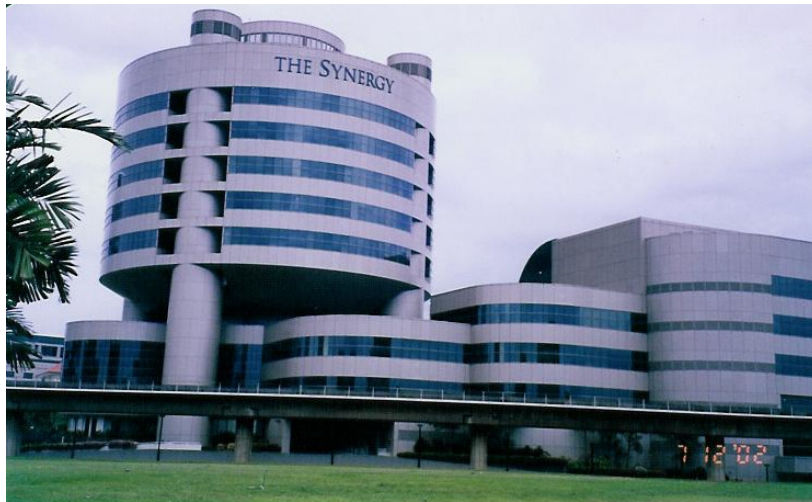
Synergy Building, Singapore
