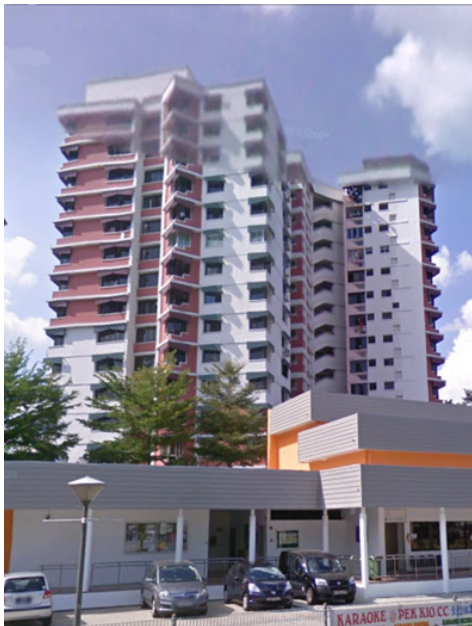
Full view of Tower Block 37
